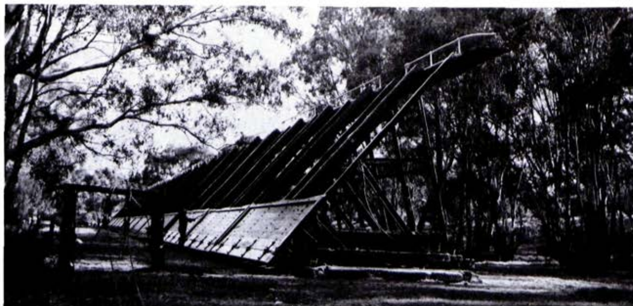
Rivers and raw materials: technical innovations, the trestle weir - Torrumbarry Weir
