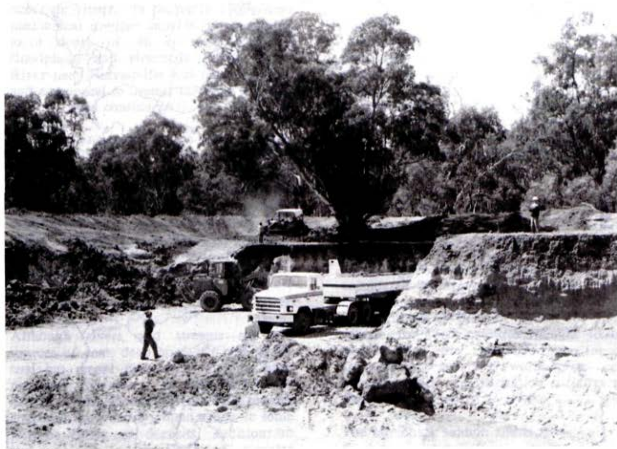
Sand extraction - Murray River floodplain
