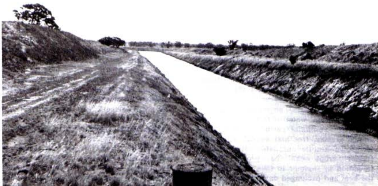
Waranga Western-Channel supplying the Goulburn--Murray Irrigation District - (Basin 5)
