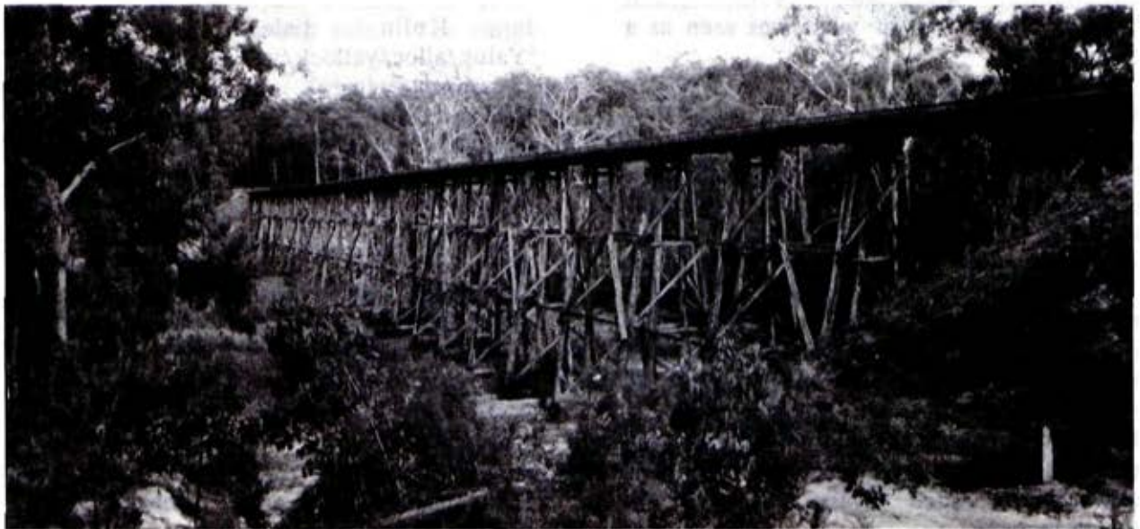
Rivers and communication: trestle bridge - Stony Creek (Basin 23)
