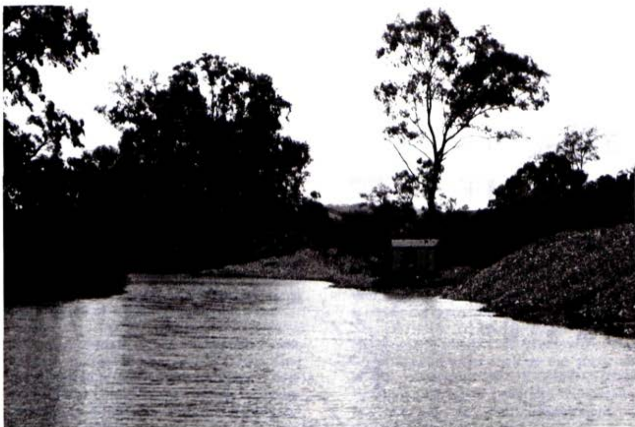
Gravel extraction - Goulburn River (Basin 5)
