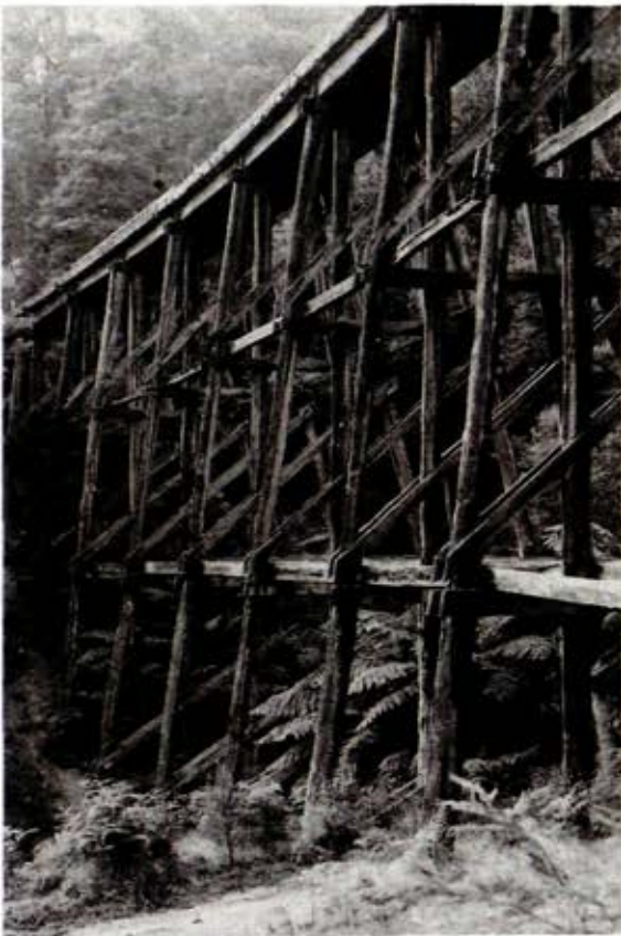
Trestle bridge on the closed Warragul to Noojee line
