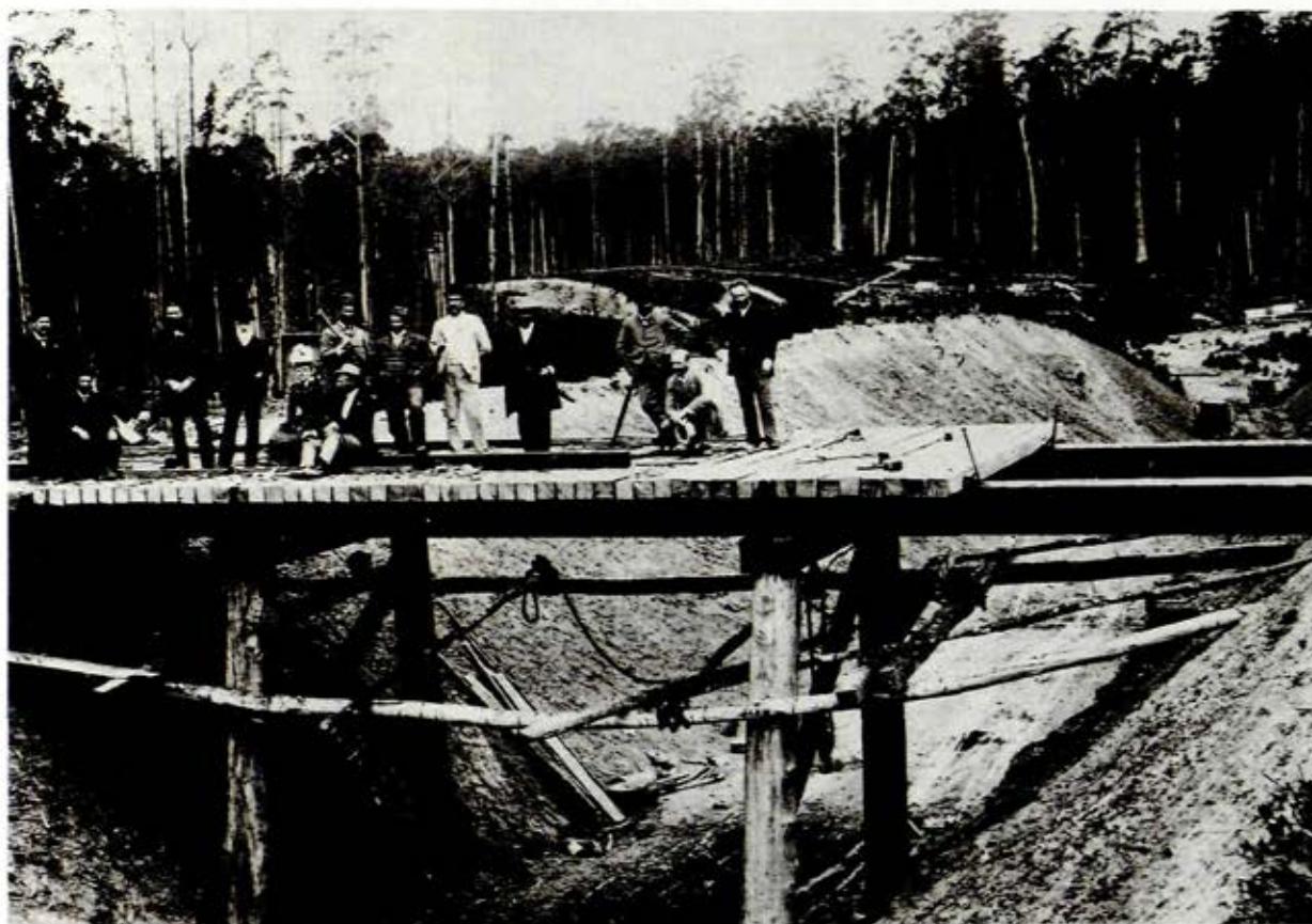
Railway construction near Korumburra
