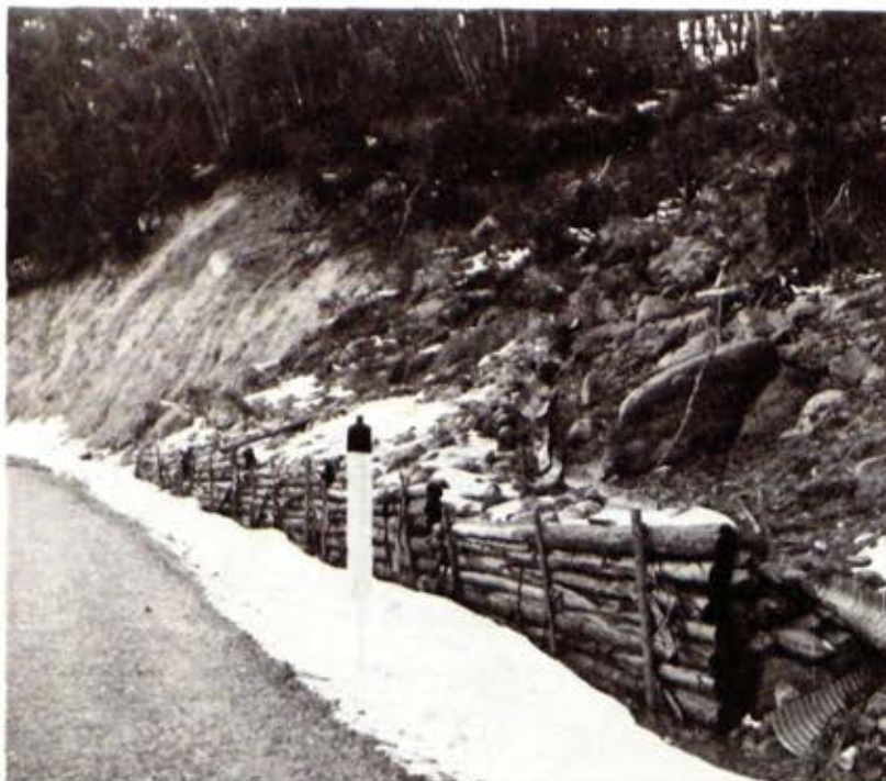
Landslip on a road in the sub-alpine zone - controlled by construction of drain and retaining wall.
