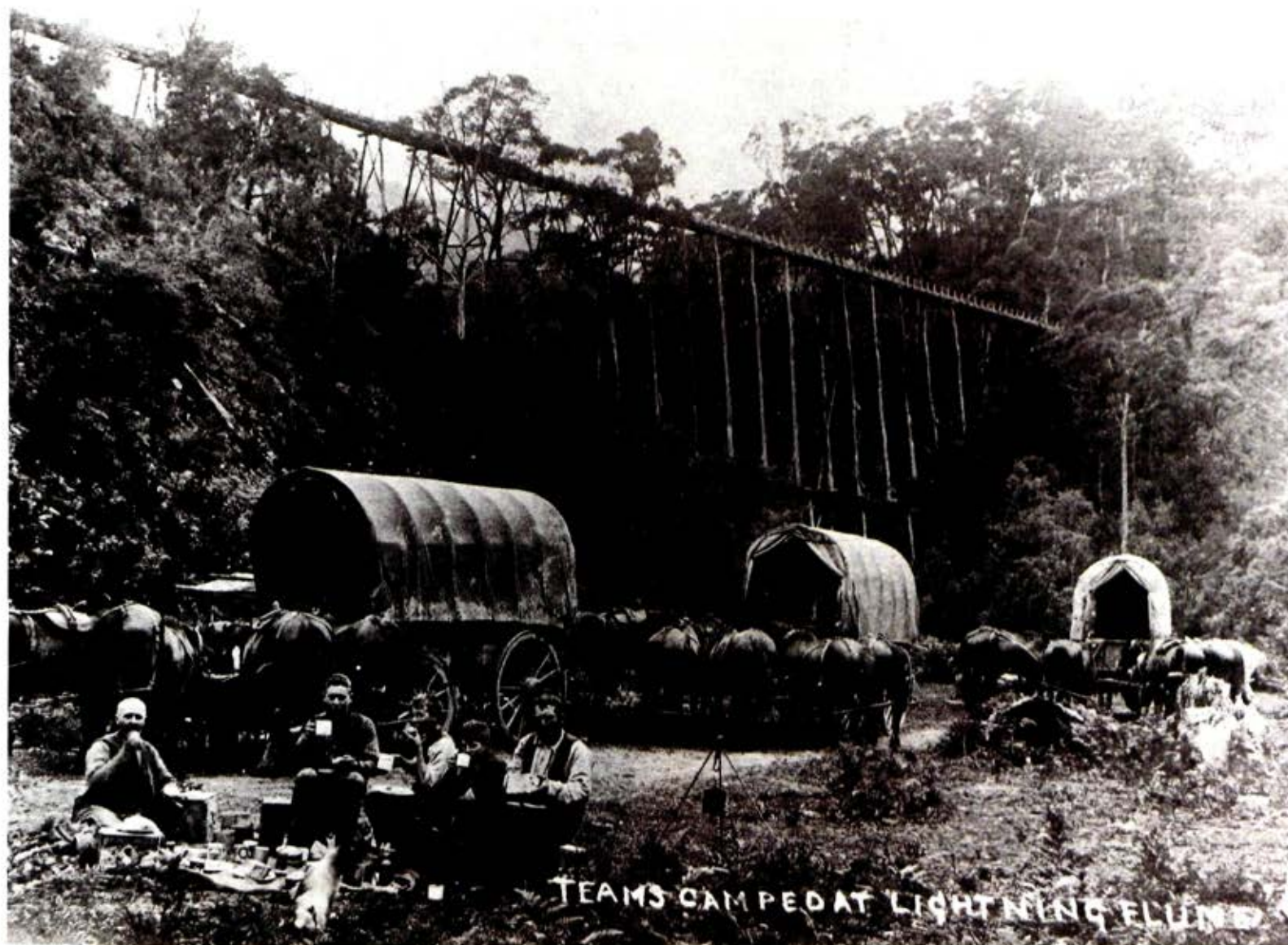
Horse teams camped near the Flume erected in 1886 to supply water for sluicing at the Mitta Mitta goldfields.
