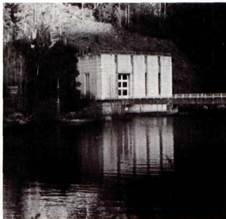
Clover power station generates electricity from water-driven turbines.
