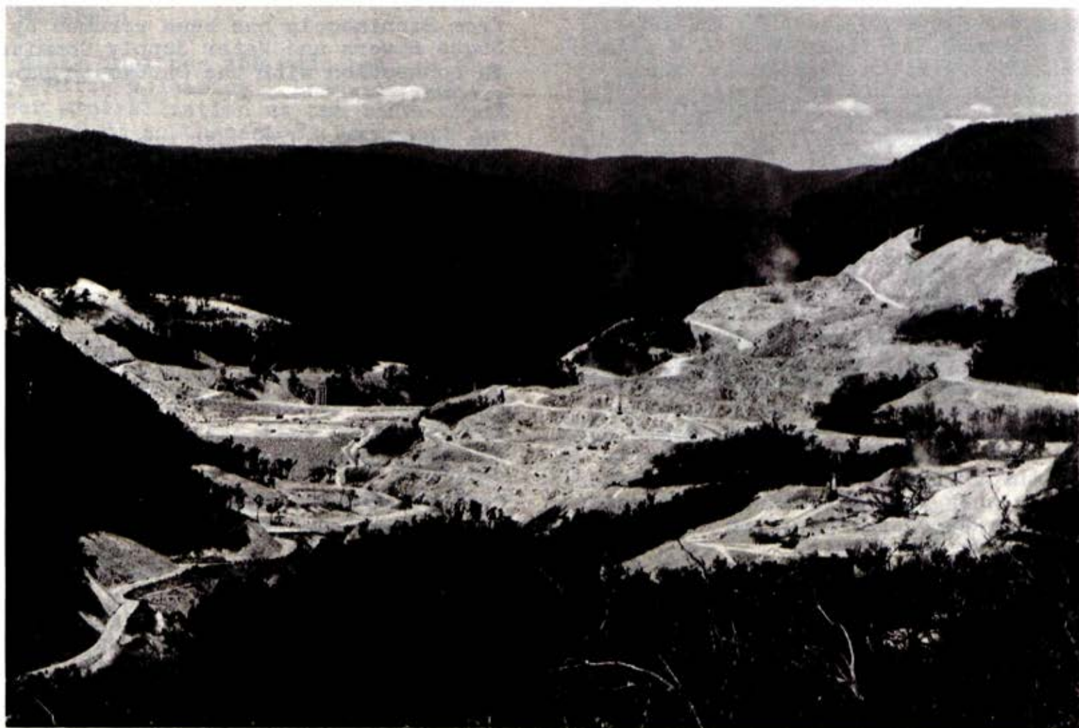
Construction of the Dartmouth Dam on the Mitta Mitta River.
