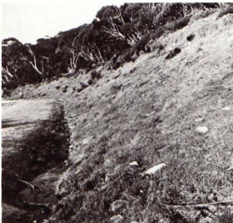
Revegetated batter slope beside this road on the Bogong High Plains helps to minimize effects of soil disturbance on the environment.
