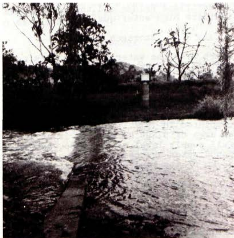
Stream-gauging station on the Tambo River at Swifts Creek.
