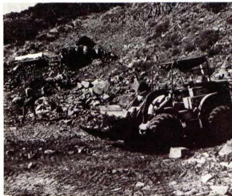
Quarrying for road-making materials.
