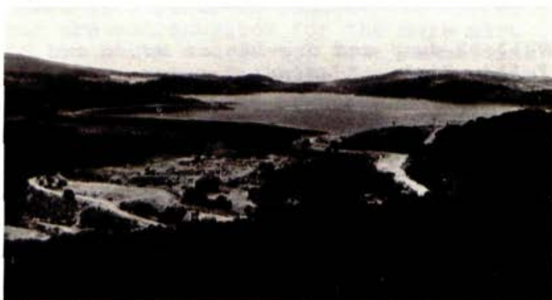
Rocky Valley pondage supplies the Kiewa hydro-electric scheme.
