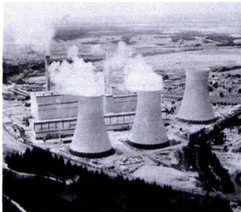
Yallourn W power station
