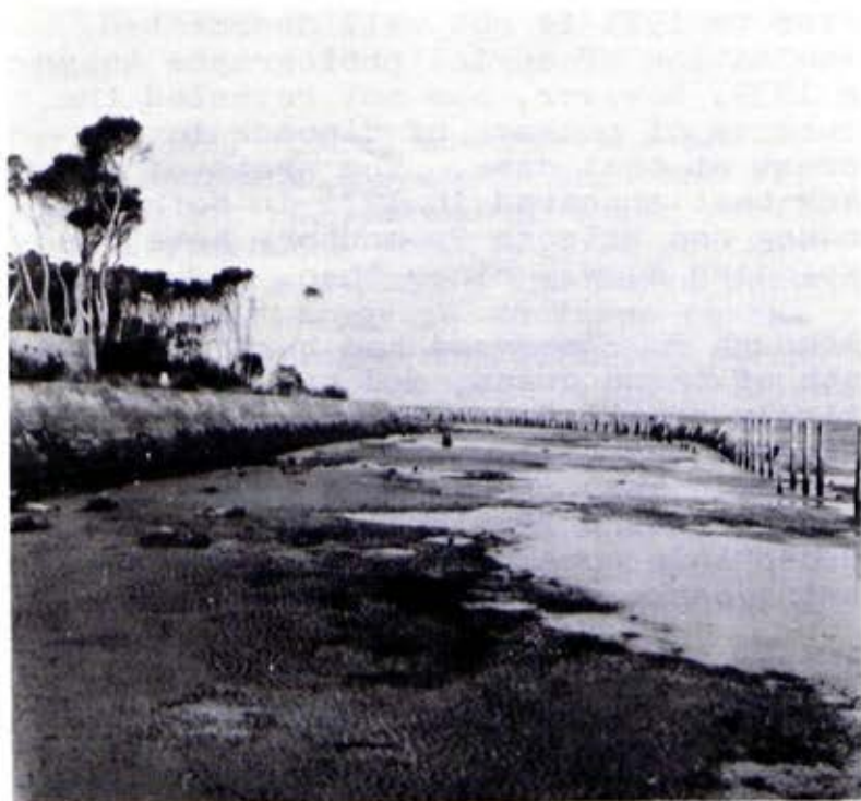
Expensive measures to protect the shoreline at Foster Beach
