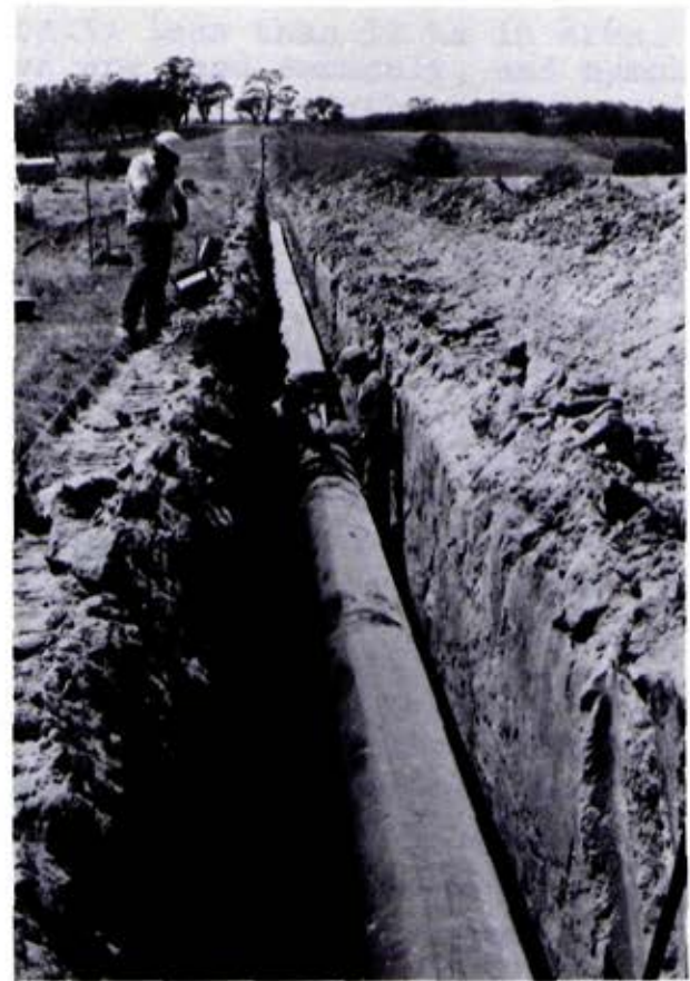
Construction of saline waste-water pipeline from Latrobe Valley coalfields to Ninety Mile Beach
