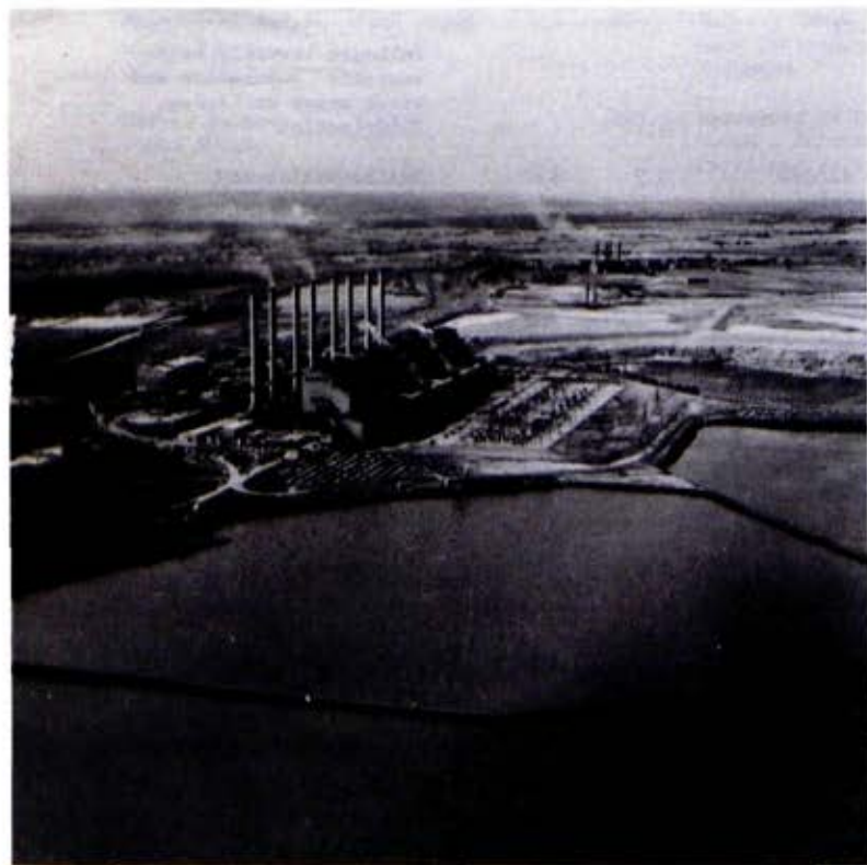
Hazelwood power station and cooling pond
