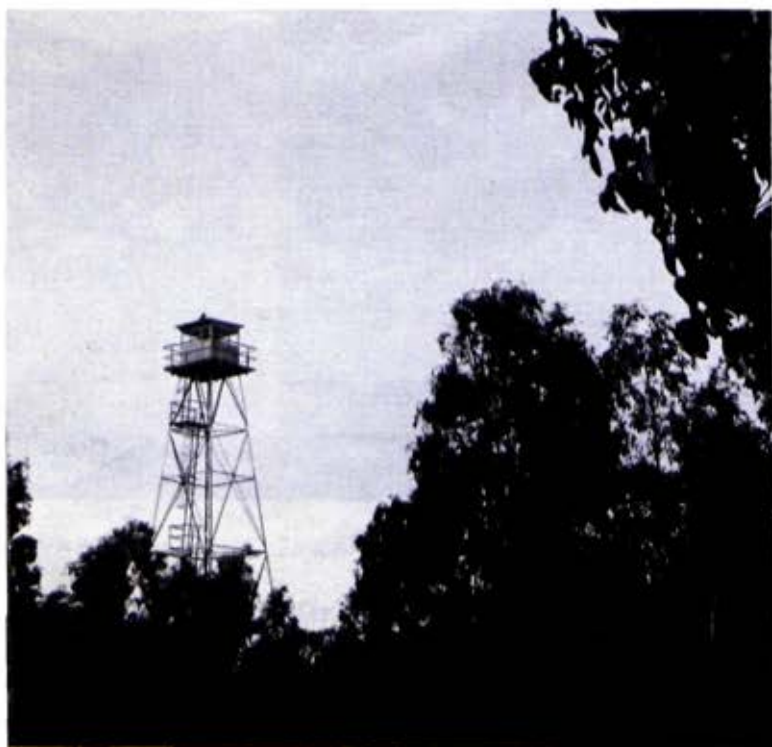
Fire tower at Dickies Hill
