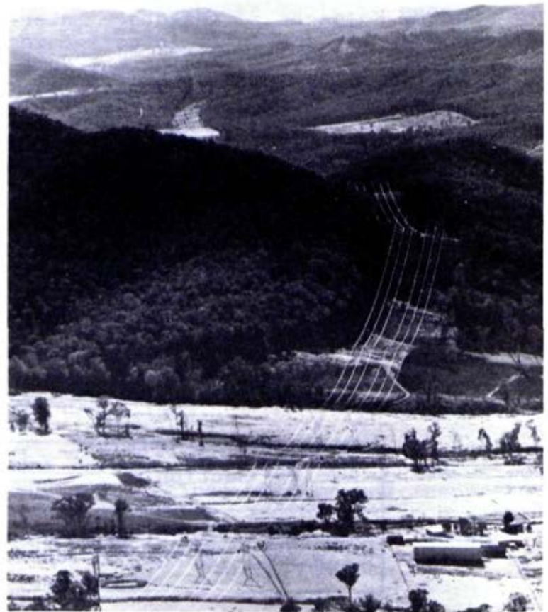
The single-circuit 330-kV transmission lines near Cheshunt
