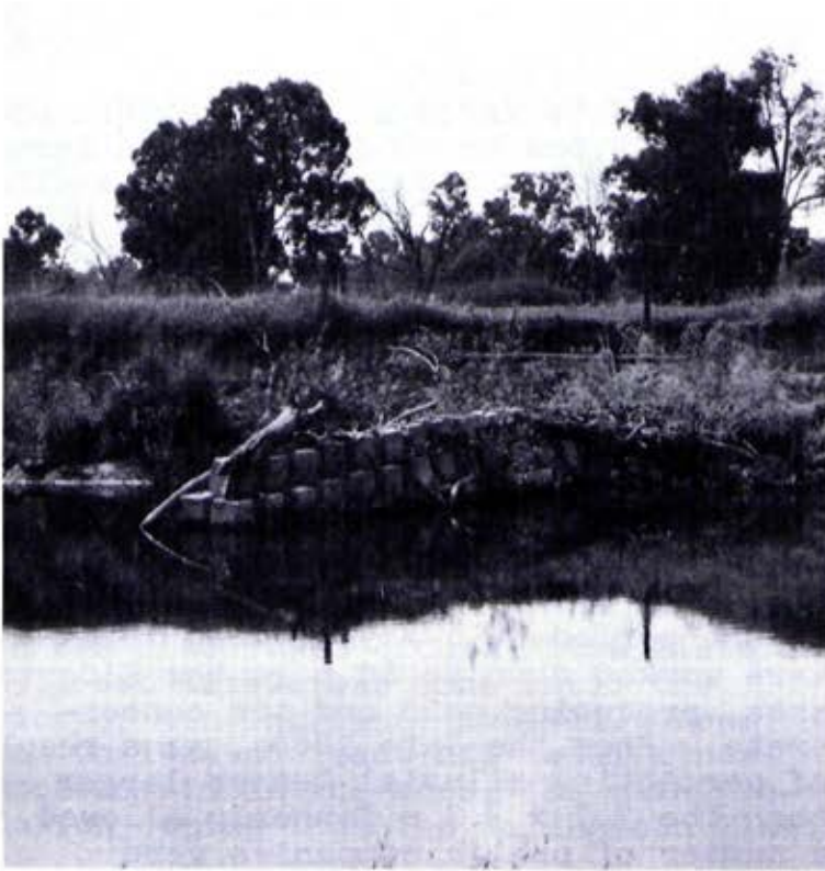
Concrete groyne to prevent bank erosion
