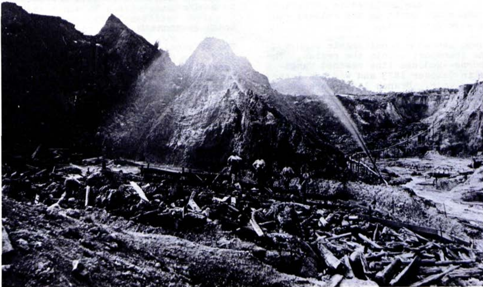
Much alluvial materials was removed by sluicing; sluicing works near Beechworth
