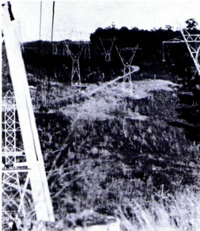
Transmission lines, although competitive with many other uses, are useful as fire breaks
