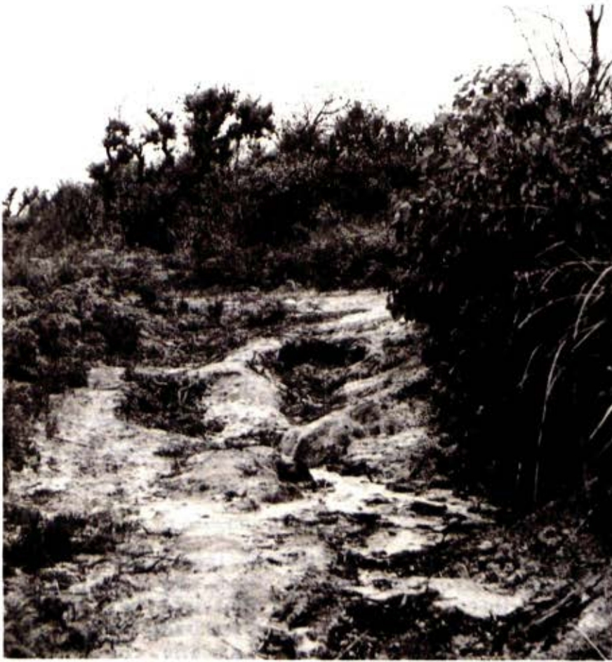
A badly eroded track on unconsolidated coastal sands
