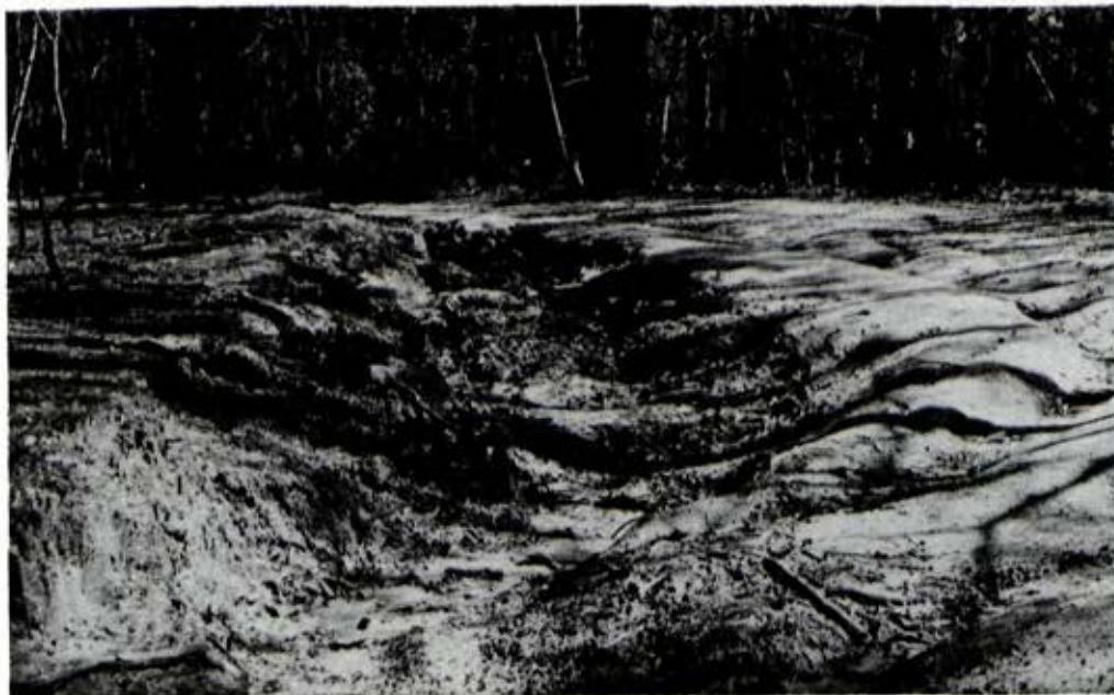
The erosion of forest tracks - such as this one north of Heyfield - is often the single most serious form of soil erosion
