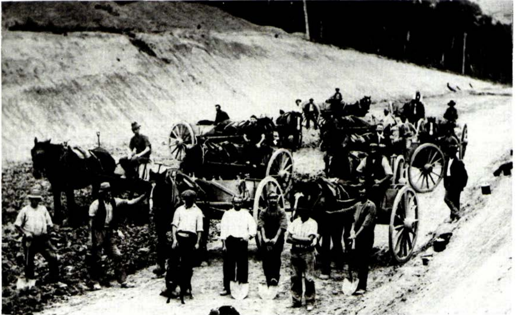
Construction gang on the Omeo Highway in the early 1900s
