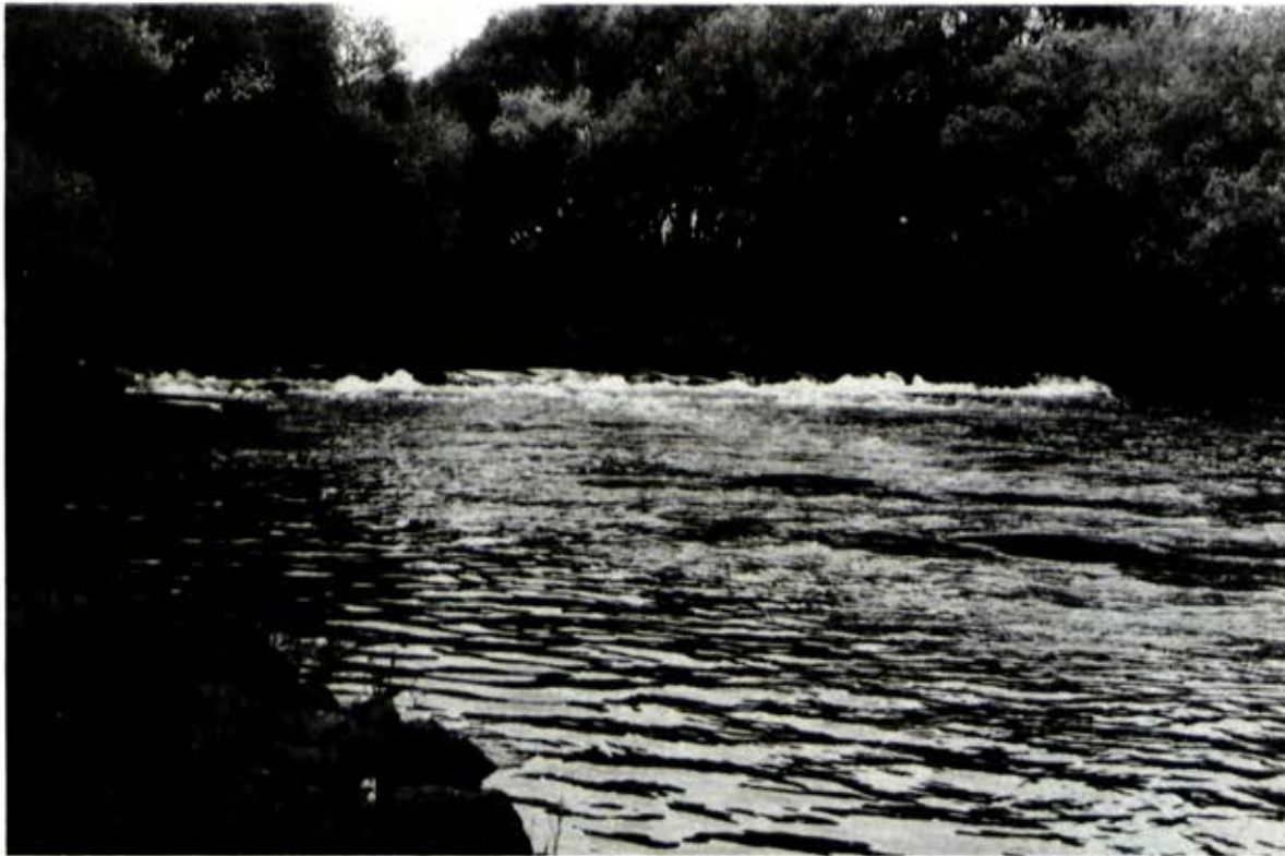
A rock barrage across the Mitchell River is designed to prevent the salt water from Lake King reaching the point where water is taken off for domestic use in Bairnsdale
