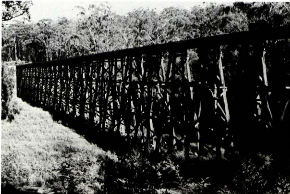
The Stony Creek railway bridge west of Nowa Nowa
