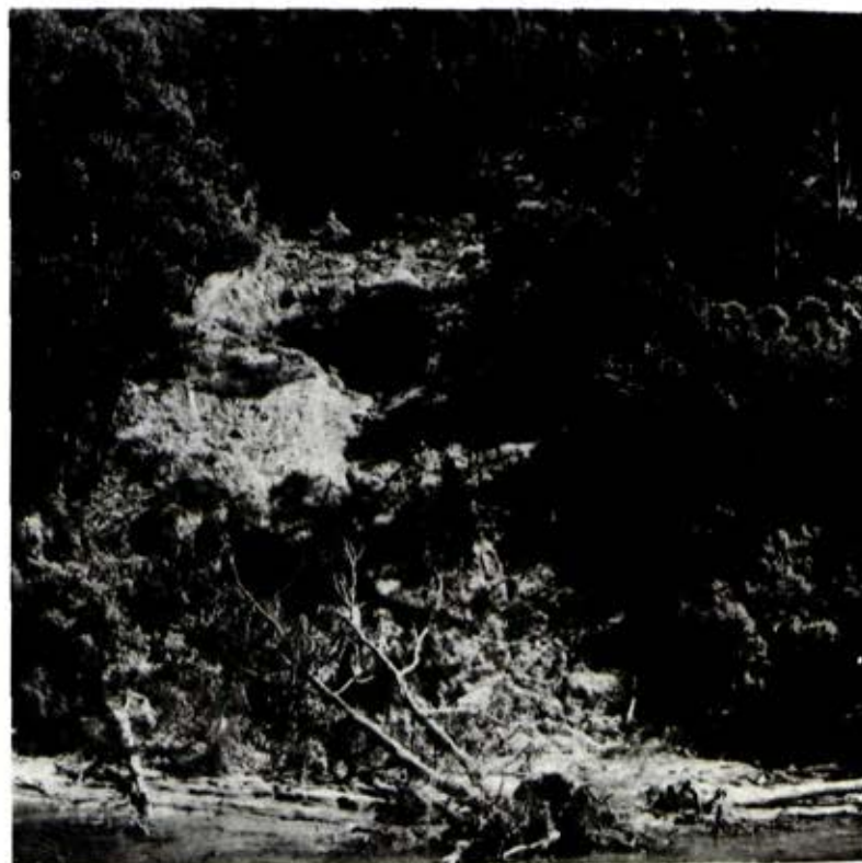
Land slips are a problem on the steep cliffs fringing the Reeve Channel between Kalimna and Nungurner
