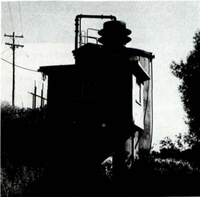
Bruthen Waterworks Trust facilities next to the Tambo River
