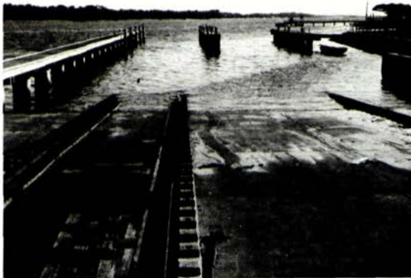
This slipway at Lakes Entrance is used for the maintenance of both commercial and recreational craft
