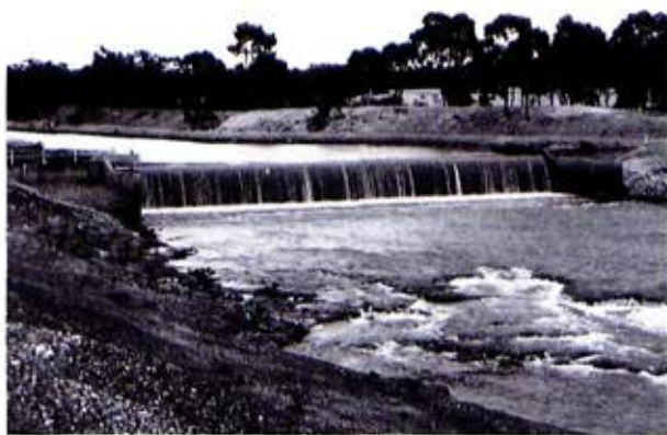
Inlet channel, Waranga Reservoir.
