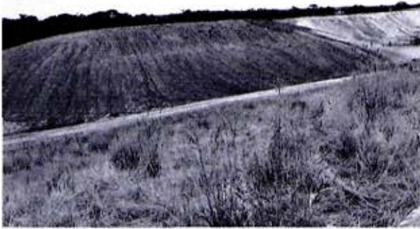
This mine tailings heap has been covered with topsoil prior to revegetation, Fosterville.
