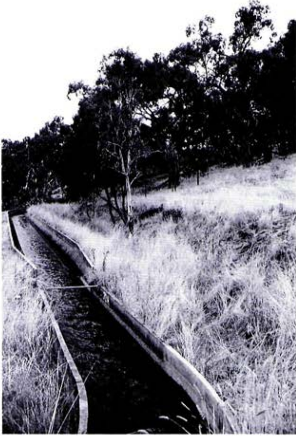
Coliban Aqueduct, north of Harcourt.
