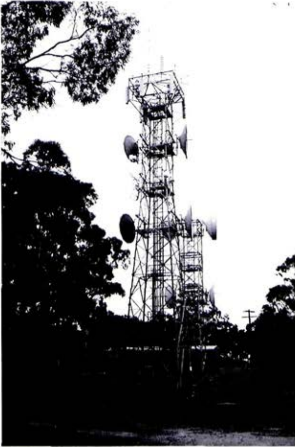
Telecommunications facility at Mt Alexander.
