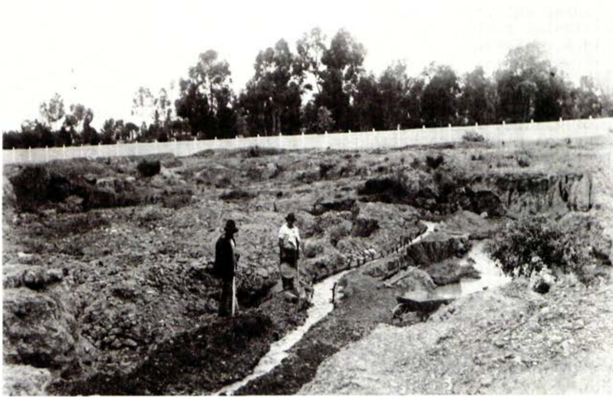
Ground sluicing
