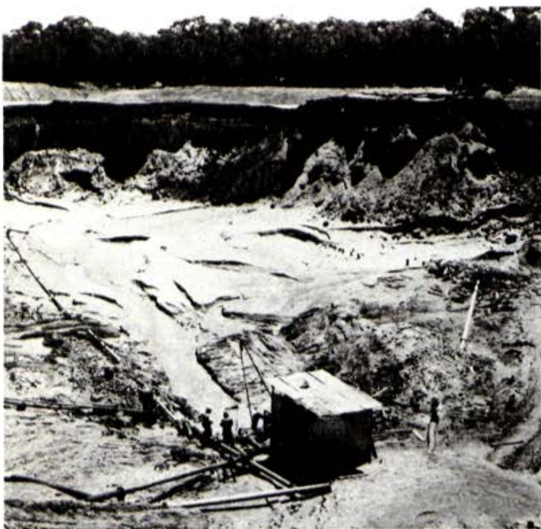
Vast area of Tertiary gravel and sand near Smythesdale. This resource is sluiced (right) and washed to produce sized sand and aggregate
