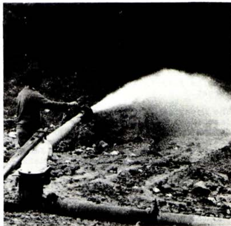
Vast area of Tertiary gravel and sand near Smythesdale. This resource is sluiced (right) and washed to produce sized sand and aggregate
