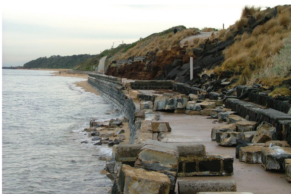
Figure 5.3 Significant storm damage to the Black Rock historic bluestone masonry seawall and promenade constructed in the 1930s is costly for land managers to repair. (Photo: M Mitchell)
