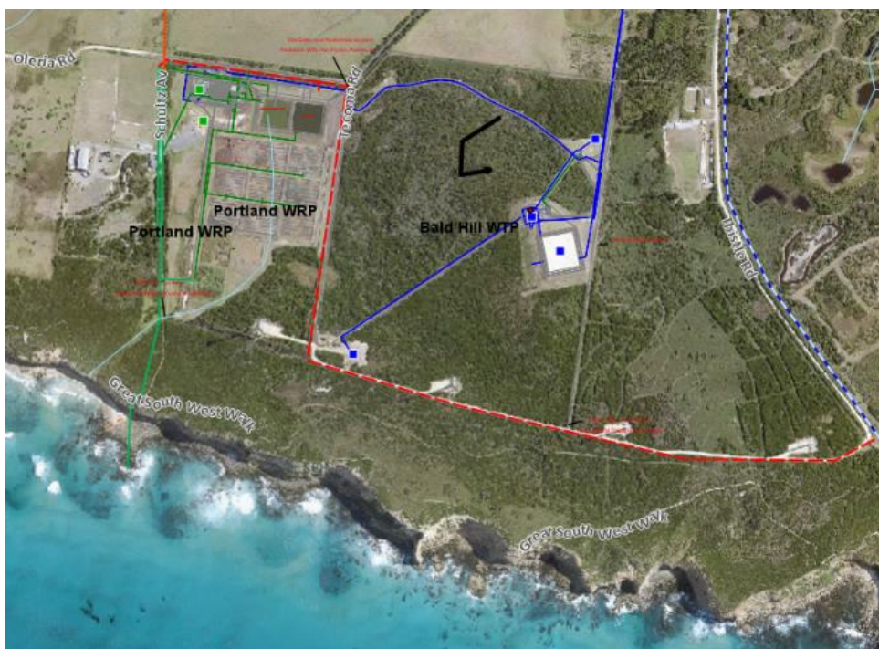
Figure 1: Portland Wastewater plant (left) and water extraction infrastructure at Bald Hill (right).
